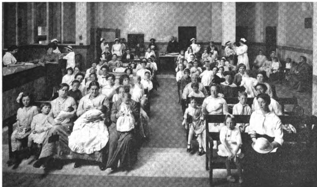
THE WAITING-ROOM IN THE NEW OUT-PATIENT DEPARTMENT AND FREE DISPENSARY, HOSPITAL FOR SICK CHILDREN, TORONTO. THE PHOTO SHOWS THE ROOM AS IT IS GENERALLY FROM 9 A.M. TO 1 P.M.
